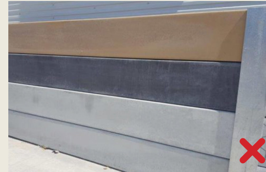
Figure 5 - Concrete Sleeper Retaining Wall
