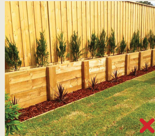
Figure 6 - Treated Pine Retaining Wall
